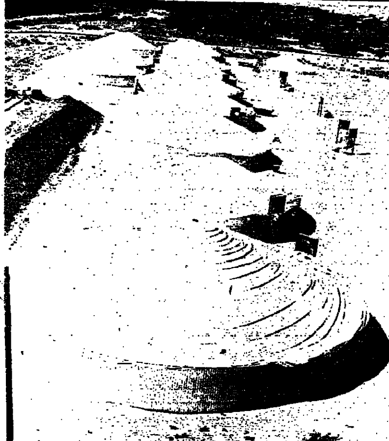
astic silos 3-4 metres high, and 30 metres in diameter. Each holds 700 tons of wheat. The ones shown are in Kiryat Gat.
